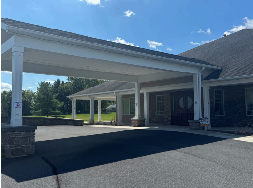
Front entrance to the temporary admin offices.
