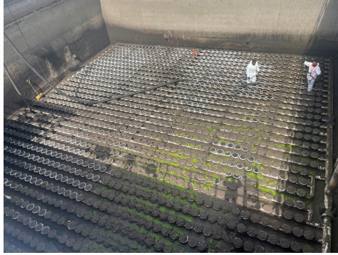
South Plant tank cleanout
